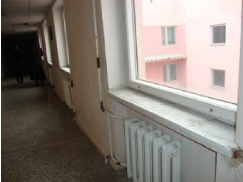
The old, single-pipe, heating-distribution system (restricted water flow)
