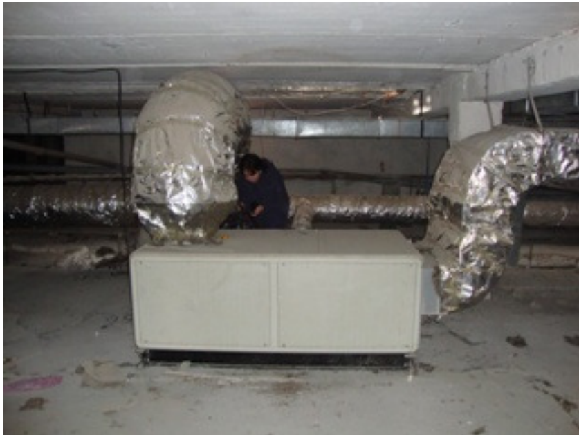
Technical floor (attic) with the air conditioner, which was never used
