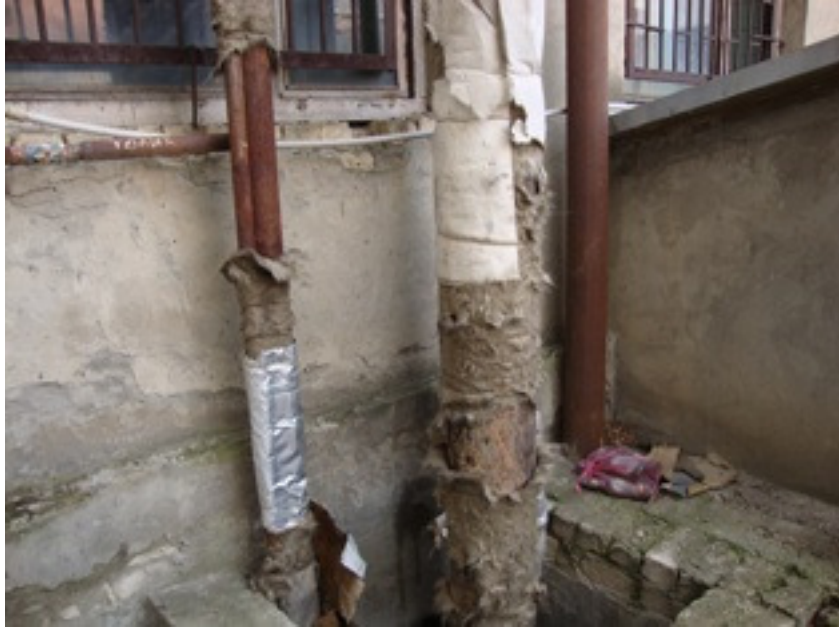
Pipelines with the damaged insulation
