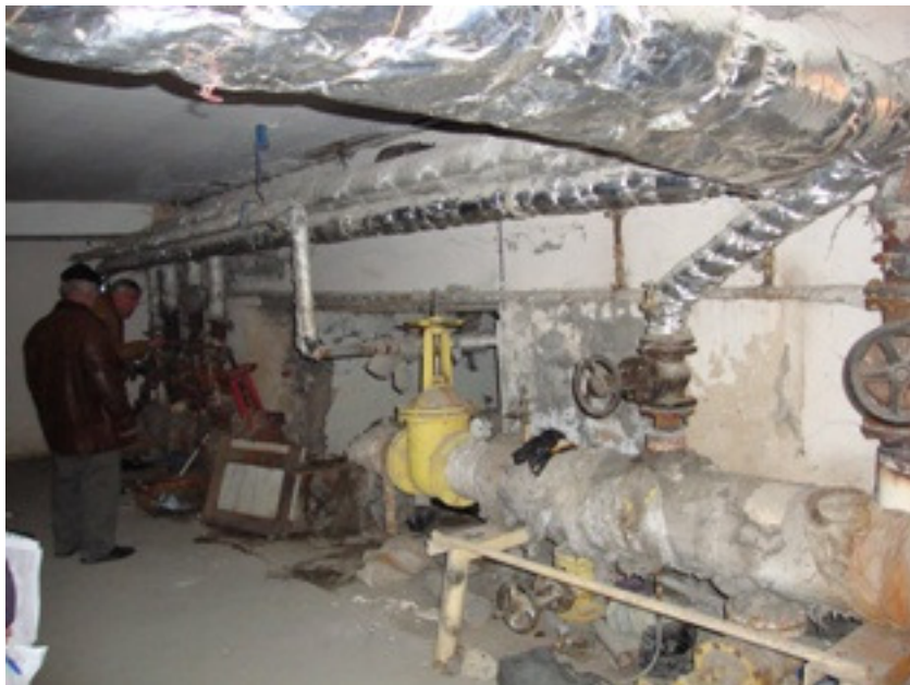
Hospital basement with the heating system main loop pipes
